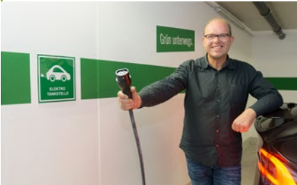
Tesla- and e-charging station
